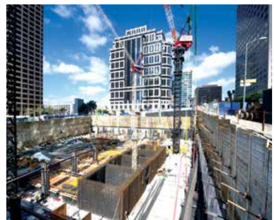
PHOTO ABOVE: The InterContinental Wilshire Grand Center under construction
