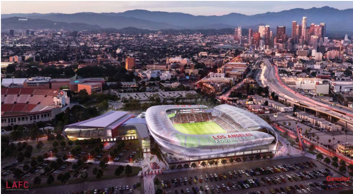
Above: Rendering of the Los Angeles Football Club stadium as viewed from the air
